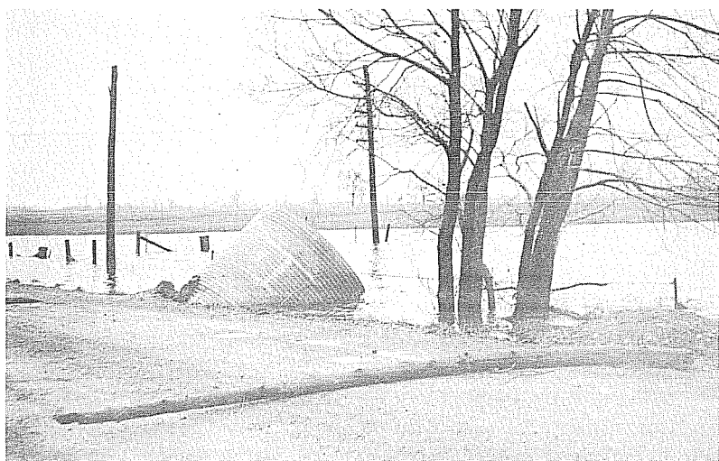
Pictures taken by Frederick Philip Grove of the actual flood on which The Adventure of Leonard Broadus was based. Taken after the waters had receded, one photo shows the water rushing over the road and the other shows the culvert which was washed up and out as the result of the pressure of the flowing water. Courtesy of Leonard Grove.
